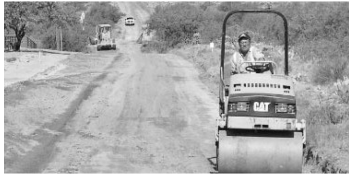
Preparing the road before Soil Sement® is applied.
