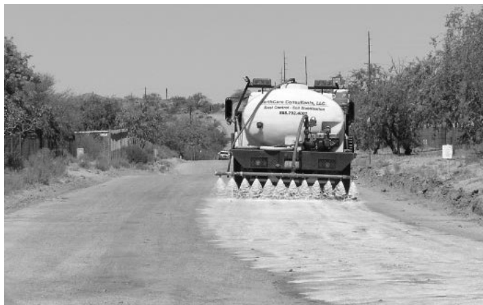
Soil Sement® being applied to Edwin Road
